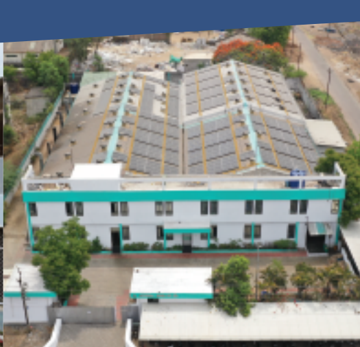
Truck Valve Plant
